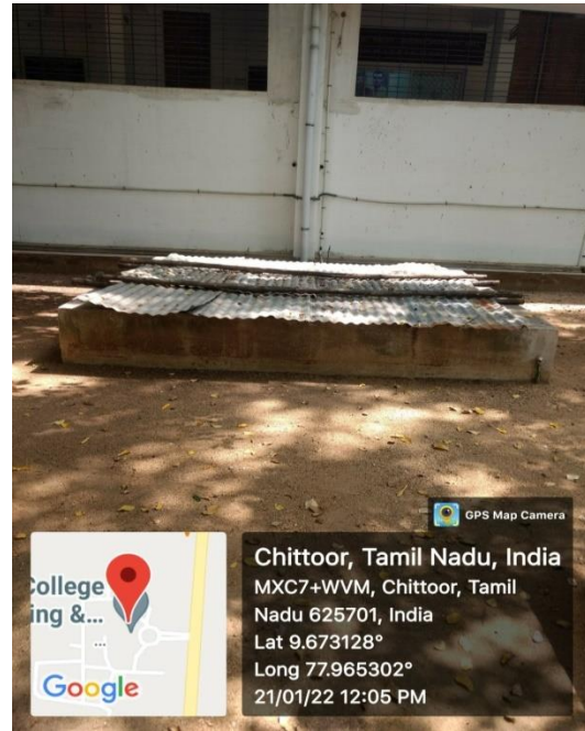
Fig. 7.1.4.2- Rainwater sumps near stores
