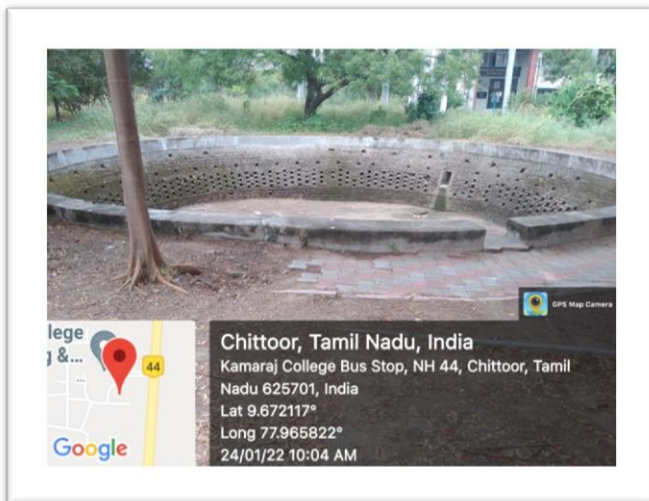
Fig7.1.4.3- Open well near power house
