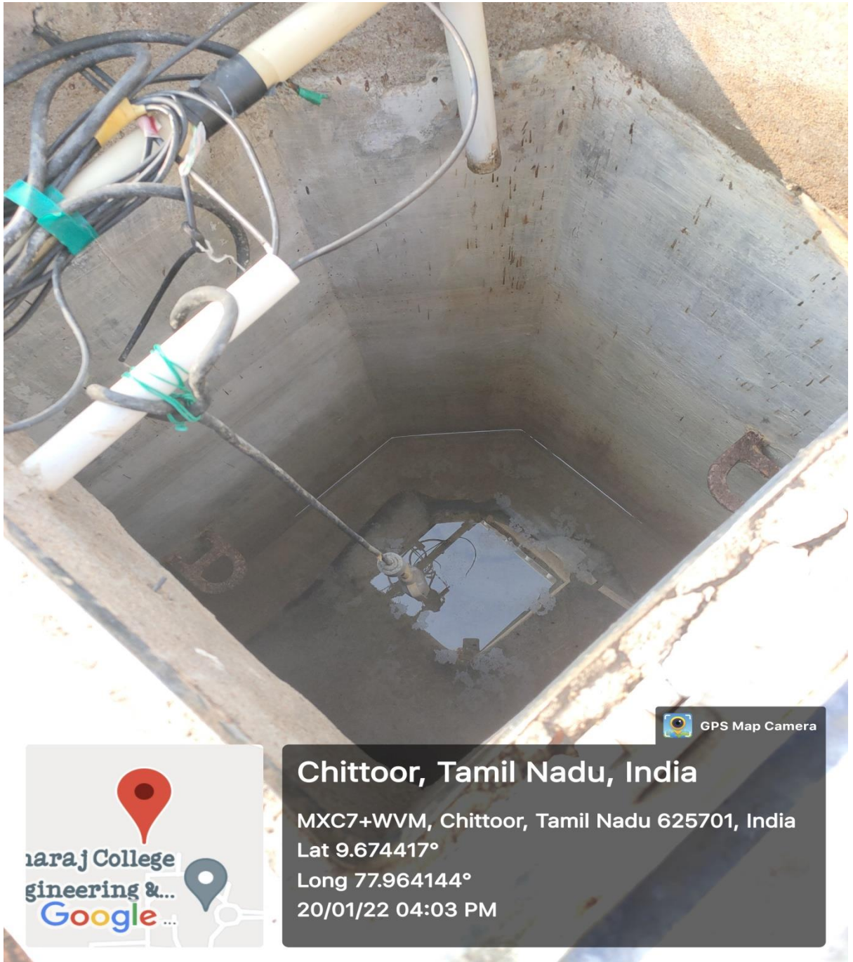
Fig: 7.1.2.6.a Float Sensors for Automatic Water Level Controller
